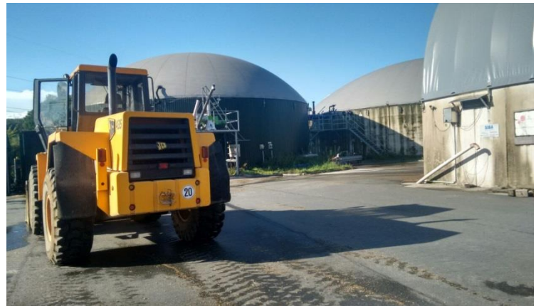
Figure 7b Biogas plant
